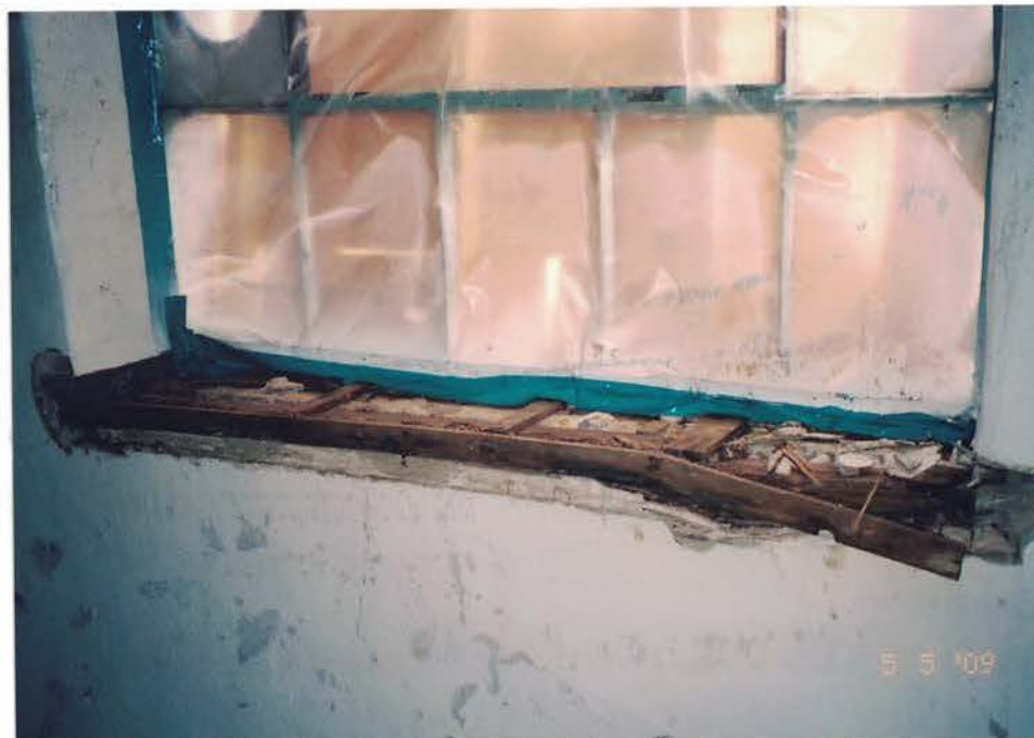
Photo #58: A LBP window sill inside the basement laundry room was removed for disposal as per the contract specifications. The LBP wooden sill is not historical, and warrants removal and disposal instead of stripping in-place. Viewing down, and to the southeast.
