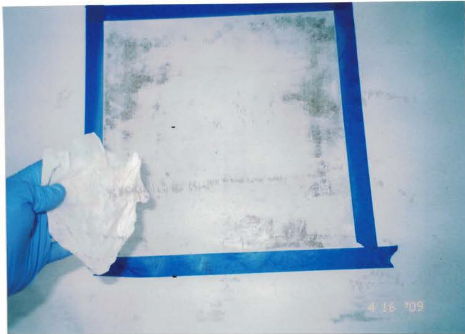
Photo #39: Post-abatement wipe sample B116-14, collected from the concrete floor inside 1st floor Room M-4, is reported with a lead content of 23 micrograms per square foot ( \text{ug}/\text{ft}^2 ) which is below the HUD clearance standard of 40 \text{ ug}/\text{ft}^2 for floors. Viewing down.
